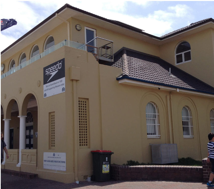
Figure 4.10: View of the north corner showing the first floor addition and the access stair to the terrace behind the parapet and the precast cement ventilation panels on the ground floor. 2015 Source: Jean Rice Architect
