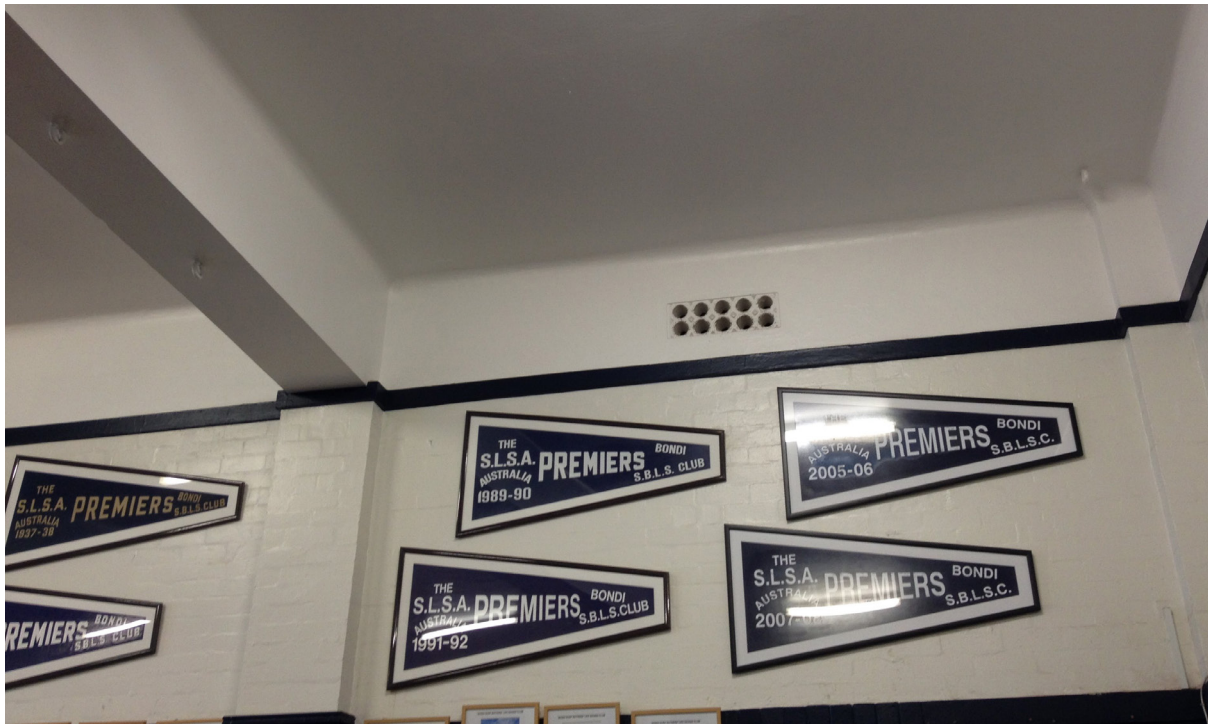
Figure 4.15: Detail of a wall vent that opens into the roofspace. Below the concrete beam the walls are face brick - now painted. Source: Jean Rice Architect
