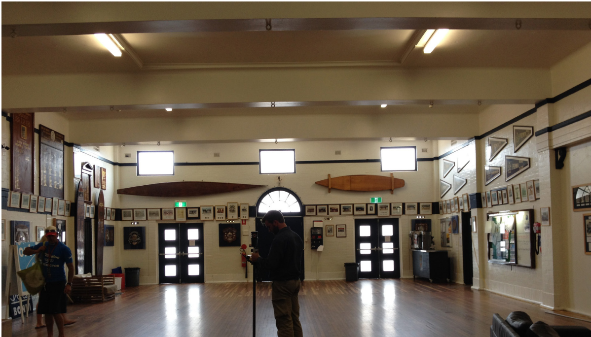
Figure 4.17: View of the central hall showing the surviving semi-circular fanlight over the front door (centre) and the three highlights above. These were originally intended to be on the sides as well but were eliminated and the, now removed, central lantern added when the design was changed to have pitched roofs on the outer side of the wall. The infilled dais is to the right. In the central bay of the ceiling, with a light on each side, is the infilled former light well / lantern location. The ceiling and beams were originally kalsomined. Source: Jean Rice Architect
