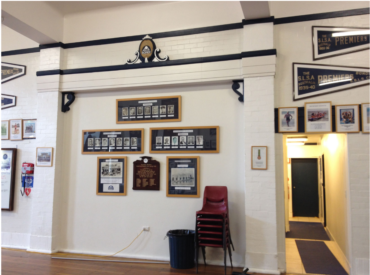
Figure 4.16: View of the infilled dais with the surf club crest over. The soldier course of bricks that forms the skirting is also visible. Source: Jean Rice Architect
